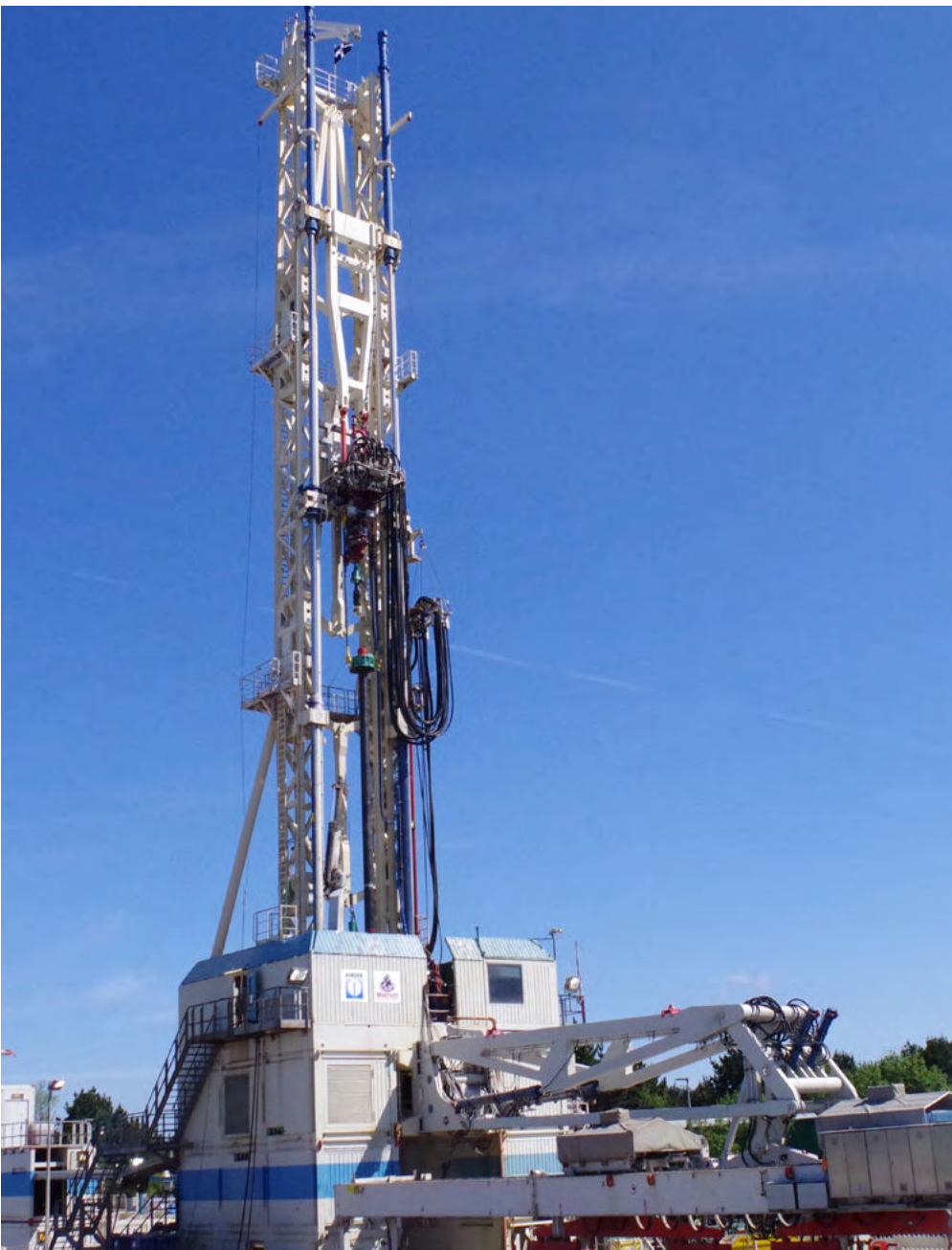
United Downs, Cornwall The United Downs project is the deepest geothermal borehole in the UK drilled to around 5.3km below ground level. This borehole utilised specialist equipment and machinery and a highly skilled team to deliver. The experience developed is directly transferable to other deep drilling projects worldwide.
